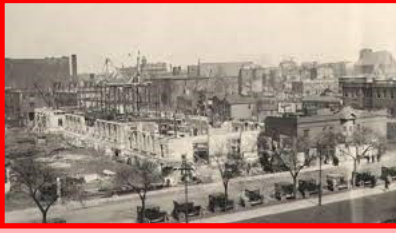
Safety Building under construction
